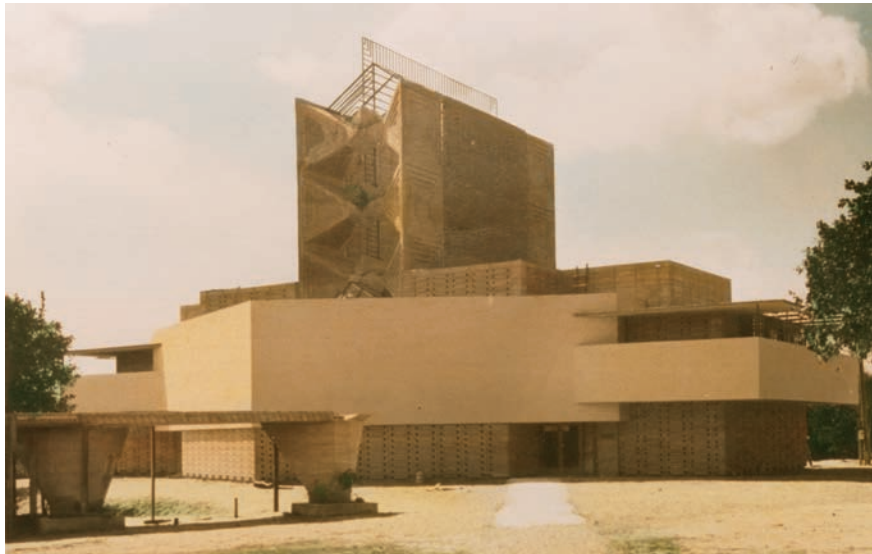
One of the earliest photos of the original Annie Pfeiffer Chapel, around 1941. Note the textile blocks extend up on either side of the base of the tower. They were later covered with stucco.
